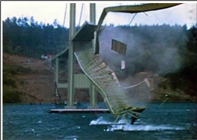
Film depicting the collapse of the Tacoma Narrows Bridge due to forced oscillatory motion. Movie from youtube . Click on image to view the movie.
